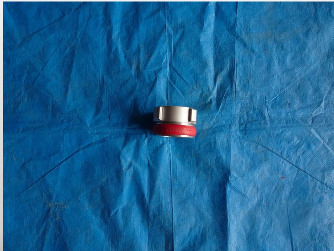
消火栓金具 (75mmメスネジ×65mm差込メス)
